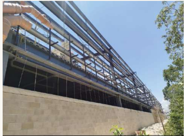
04 • Structural steel and roof erection
