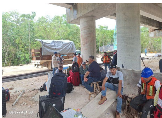
Construction personnel at the viaduct work front.
