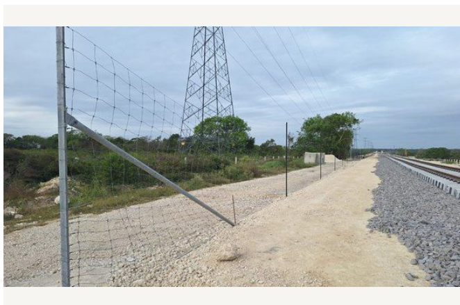
Perimeter enclosure alongside the railway.
