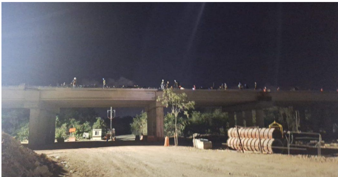
Night work on the elevated viaduct.
