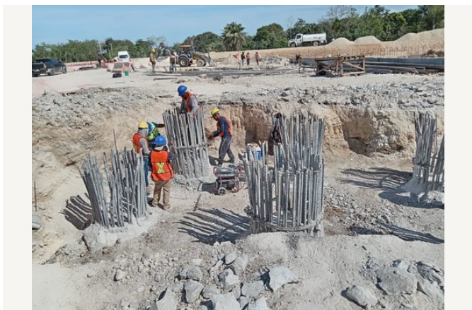
Works on deep foundation elements.
