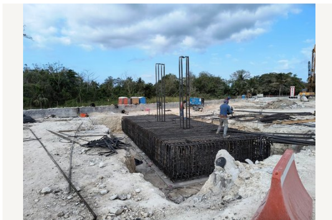
Assembly of foundation reinforcement.
