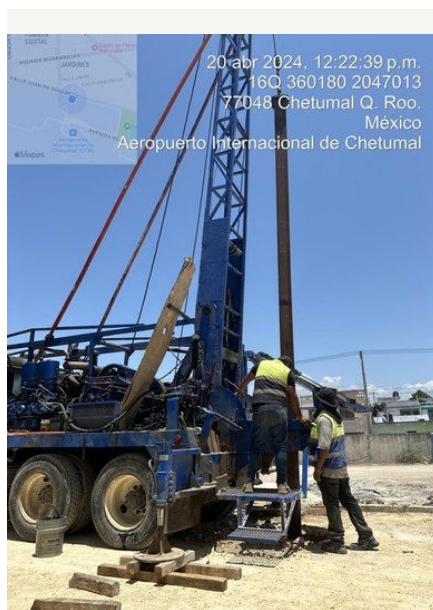
Drilling with truck-mounted equipment.
