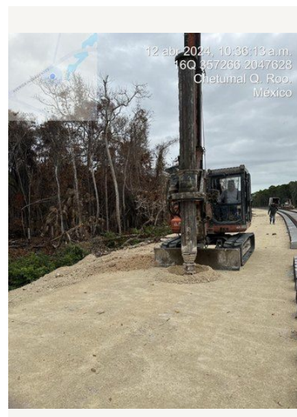
Drilling with crawler-mounted equipment.
