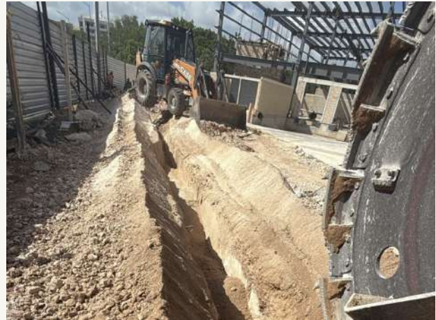
02 • Earthworks and high-capacity trenching
