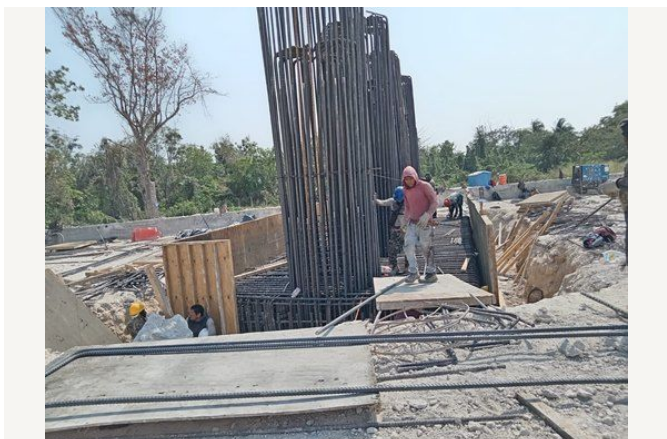
Formwork for foundation elements.
