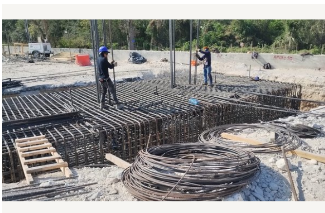
Reinforcing steel fabrication.
